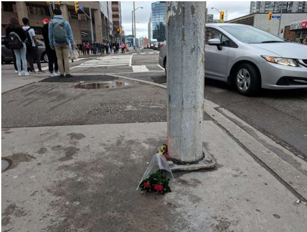
Figure 4 - Factors that increase soft target risk, zero level change on curb separating the sidewalk and street, situation facilitates easy driving onto sidewalk, corner of Yonge and Finch in Toronto, location where van attack started, depicted on one-year anniversary of van attack on April 23, 2019. Photo by Jack Rozdilsky.
