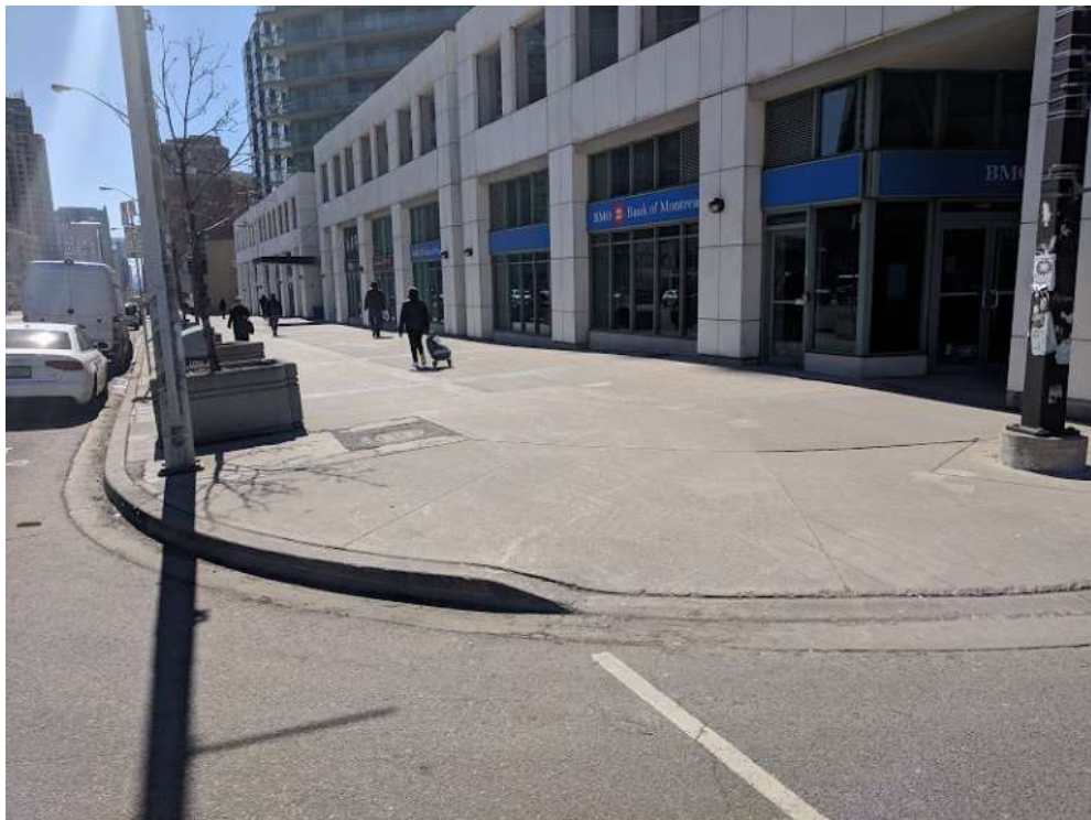
Figure 5 - Factors that increase soft target risk, view along van attack path at a barrier free corner location where a would-be attacker could easily drive onto the sidewalk, Yonge Street Toronto, depicted on March 26, 2019. Photo by Jack Rozdilsky.
