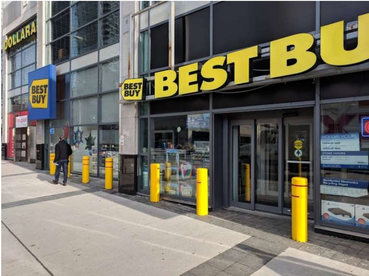
Figure 8 - Soft target risk reduction example, Cement bollards act to protect this storefront from vehicular attack, but while the building is protected pedestrians remain exposed, Yonge Street Toronto, depicted on November 29, 2018. Photo by Jack Rozdilsky.
